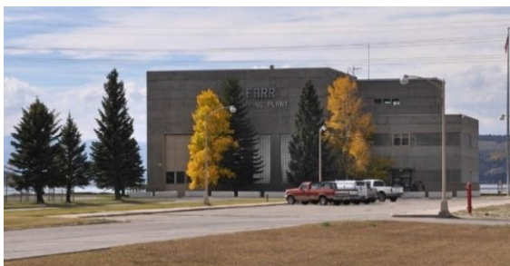
Farr Pump Plant
