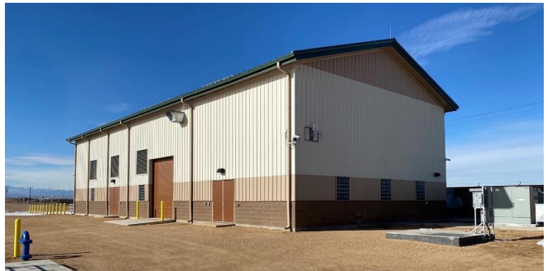
The Eastern Pump Plant neared completion in 2021.
